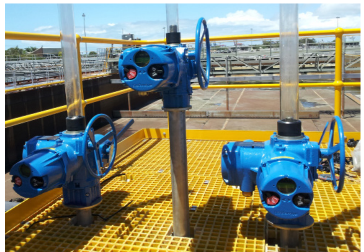
After Limitorque Slug Draw Off Upgrade
